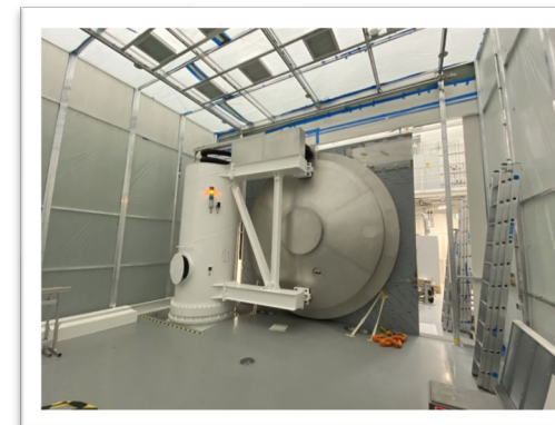
cleaning & leak check
